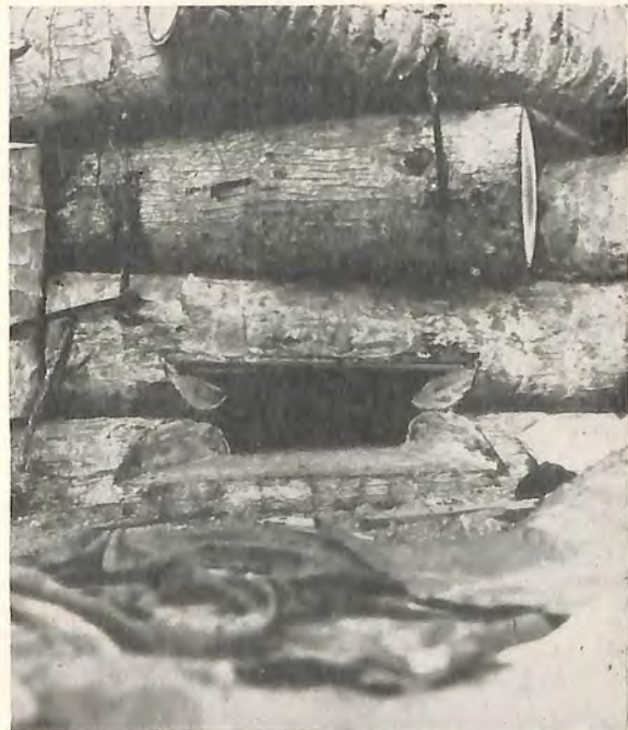
Figure 141. Front view of a pillbox.
